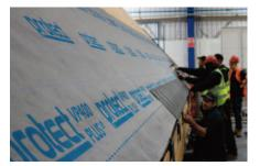
Protect GDB10 Plus - Glidevale's universal barrier membrane was used to provide enhanced ground gas and damp protection. The membrane's resilient, high puncture resistance eliminated the risk of tearing upon application.
