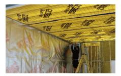
**Protect sealing tapes** – these were used with the above construction membranes to ensure correct detailing in the sealing of overlaps to significantly reduce air leakage and therefore keep energy consumption to a minimum.
