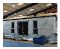
Protect VC Foil Ultra – this reflective and low emissivity air and vapour control layer was used on the warm side of the insulation within an unventilated cavity. Combined with Protect TF200 Thermo, this helped the structure achieve its target thermal performance.
