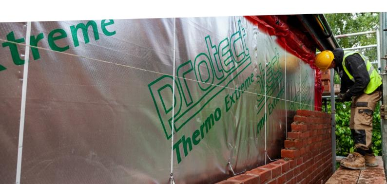
By using a fabric first approach, we combined Glidevale Protect's high performance, reflective membrane for external walls with an internal airtightness and vapour control layer. This helped to improve thermal efficiency and ensure low U-values, contributing to a low ecological footprint on each home and putting One Manchester at the forefront of sustainability.
