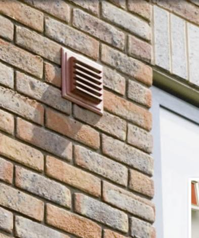
he Glidevale range of Fresh wall ventilators has been specifically designed to introduce fresh air into our homes in order to control condensation, and being non-electrical they use no energy to operate. The vents direct the air flow from around the centre of the room to effectively disperse it.
