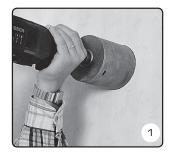
Use a core drill with min. dimension Ø102mm for Fresh 90 and Ø 150mm for Fresh 90dB. Drill from inside to outside. Drill the hole so that the pipe slopes slightly downwards.
