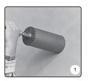
Use a core drill with min. dimension Ø102mm for Fresh 100 and Ø150mm for Fresh 100dB. Drill from inside to outside. Drill the hole so that the pipe slopes slightly downwards.
