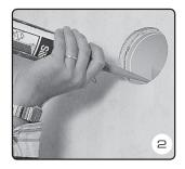
Mount the pipe and seal against the wall, both inside and outside, with for example a sealing agent.
