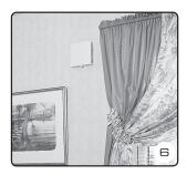
Attach the front cover. The vent is now completely installed.
