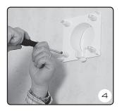
Attach the internal vent housing with 4 screws.
