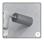
Use a core drill with min. dimension Ø86mm for Fresh 80 and Ø 150mm for Fresh 80dB. Drill from inside to outside. Drill the hole so that the pipe slopes slightly downwards.
