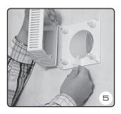
Place the internal butterfly vent arm in the slot.
