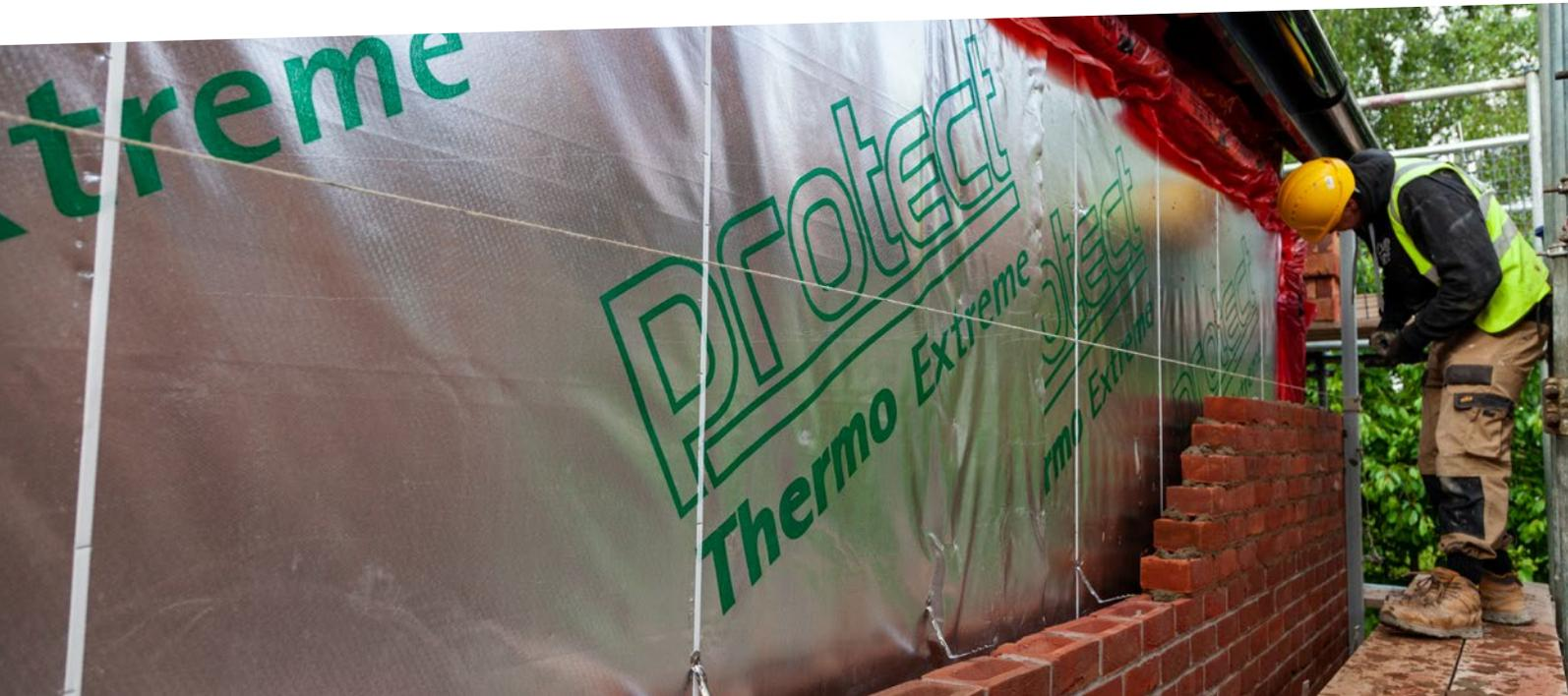
By using a fabric first approach, we combined Glidevale Protect's high performance, reflective membrane for external walls with an internal airtightness and vapour control layer.
