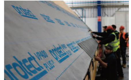
**Protect GDB10 Plus** - Glidevale's universal barrier membrane was used to provide enhanced ground gas and damp protection. The membrane's resilient, high puncture resistance eliminated the risk of tearing upon application.
